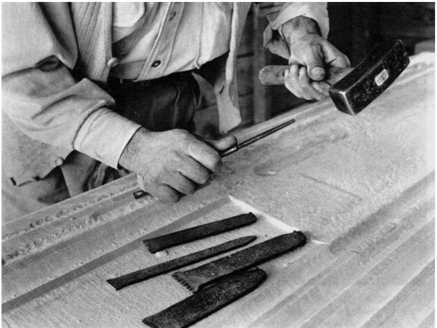
19. CHANNELING A COLUMN OF THE UPPER FRONT ORDER. In this series, in which the shaft was a single piece of marble, the channeling was done before setting. The marble worker's tools have changed little since ancient times.
