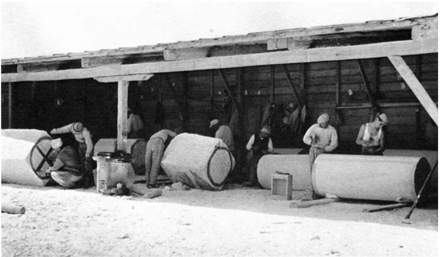
18. CARVING COLUMN DRUMS. The blocks as delivered from the quarry were roughly squared. The four corners were then chamfered, and soon the block became a cylinder. All this work was done by hand in the shelter of simple sheds: primitive stoas.
