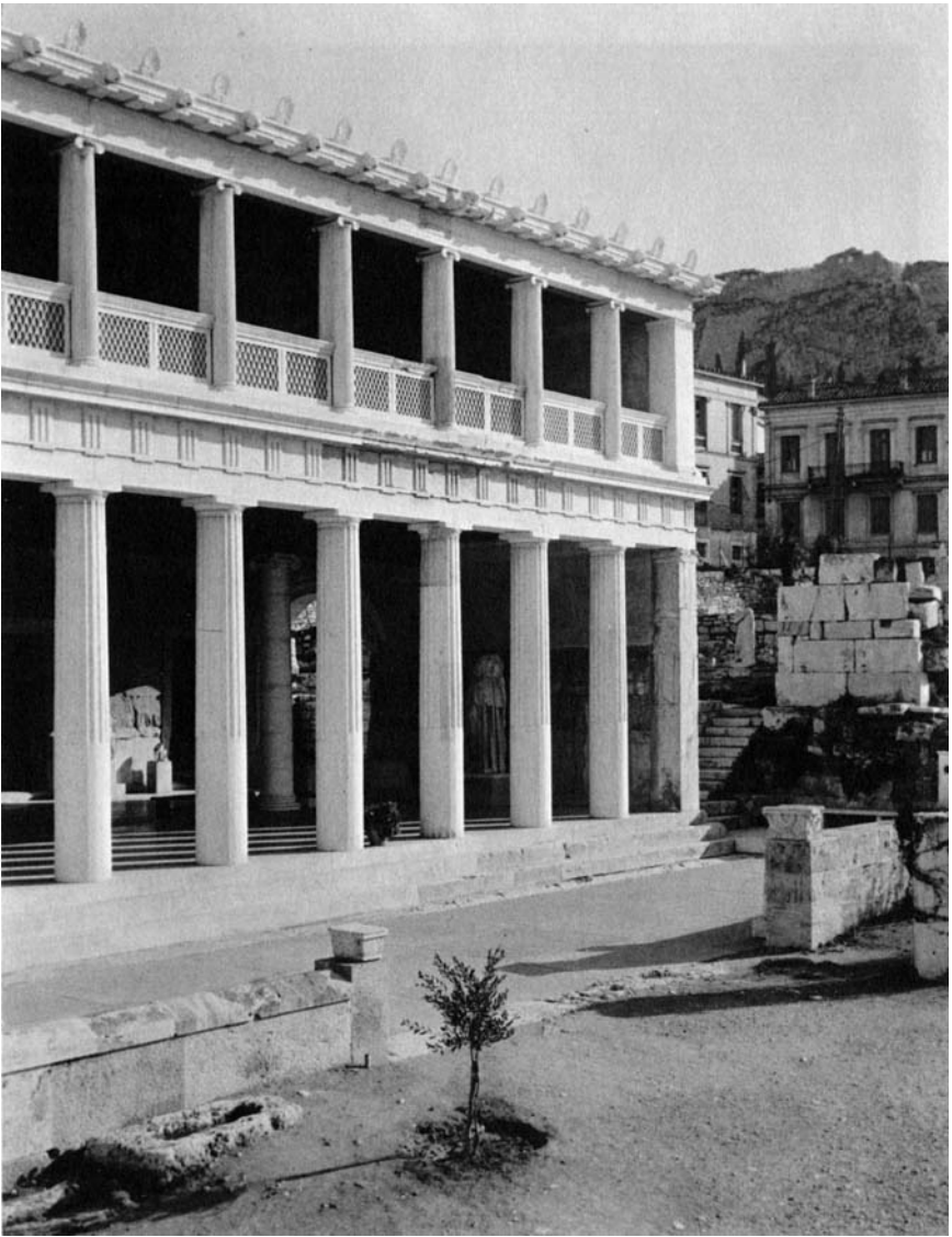
4. OLD AND NEW IN THE FAÇADE OF THE STOA. Toward the south end of the building the ancient marble steps had survived, as also much of the wall and the square corner pier. In the reconstruction of this part of the façade representative pieces of the ancient architectural members were incorporated in the new marble to indicate the evidence on which the reconstruction is based.
