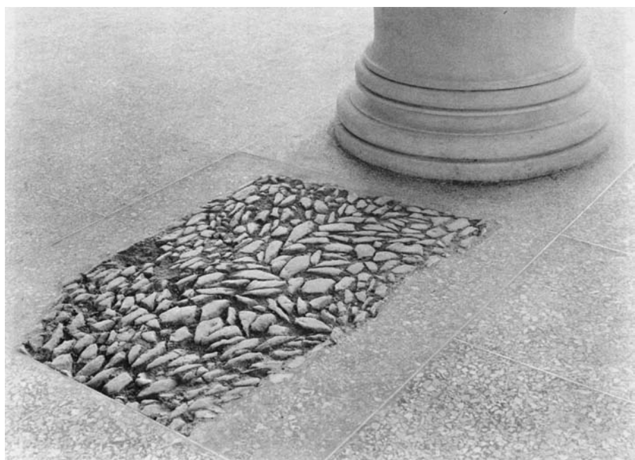
21. FLOORING. In the north end of the building a few patches of original floor were found: a rough mosaic made of marble chips imbedded in lime mortar. The new floor likewise consists of chips of marble (and some of limestone) rolled into mortar and polished.
